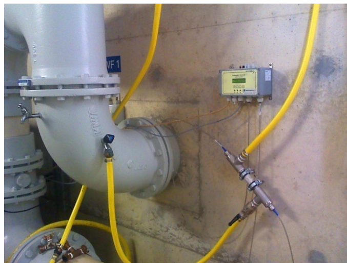
Simple installation. A Kemtrak DCP007 photometer with a long pass flowcell
